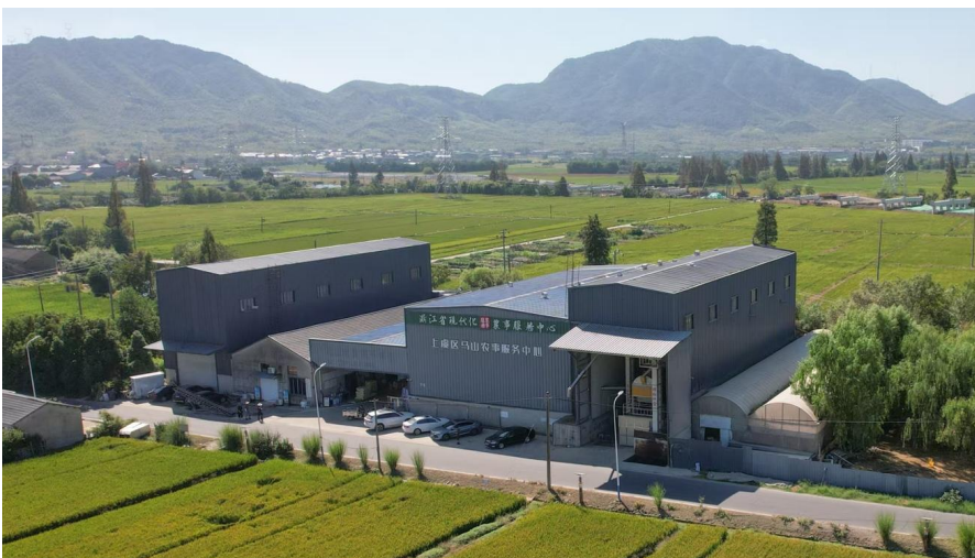
Figure 1 Aerial view of Mashan Agricultural Service Center and surrounding paddy landscape (Photoed by Xinfeng Ren)
